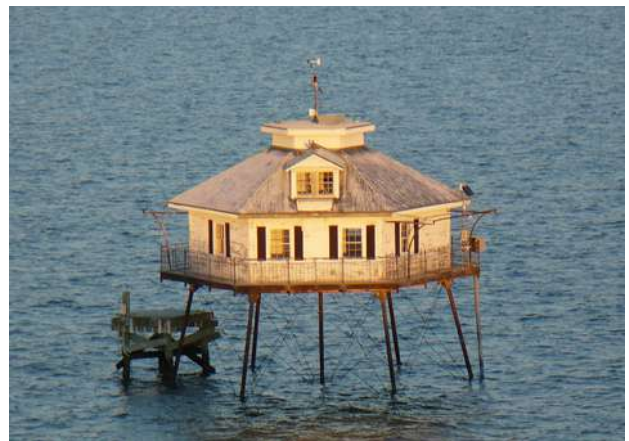
View of the Middle Bay Lighthouse in Mobile Bay, Alabama, 2008, taken from aboard the MS Holiday by Altairisfar .
